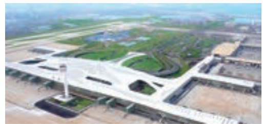
Wuhan Tianhe International Airport
